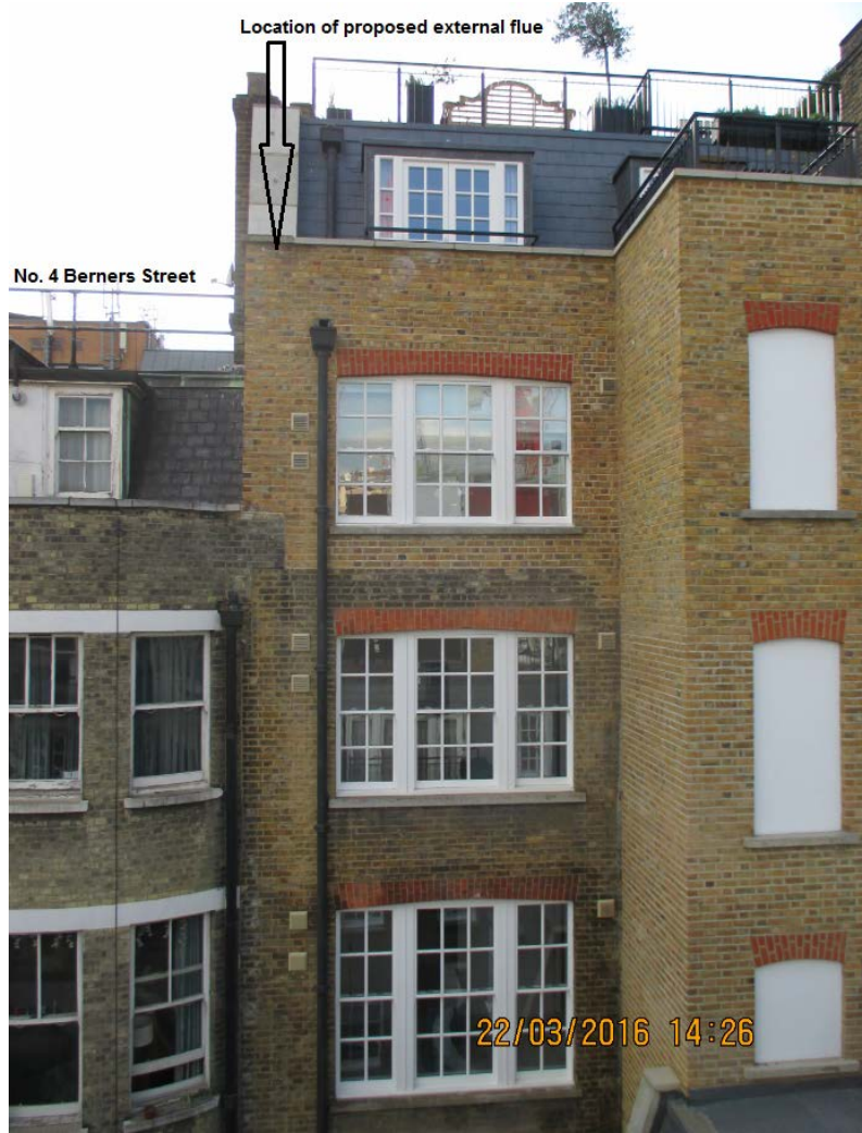
Photograph 1- Rear elevation of 5 Berners Street
